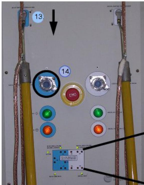
13. At the Enclosure Door/High Voltage interlock panel insert the manual grounding rods in to the key-slot and slide them downward to lock the corresponding doors.
