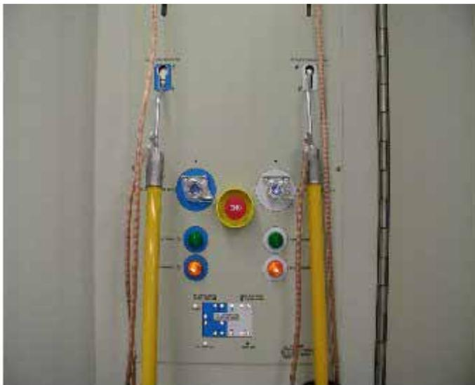
**Note:** Each grounding rod fits into a color coded receptacle. The left side is color coded blue and corresponds to the 40 KV enclosure doors 1, 2, 3, and 4. The right side is color coded white and corresponds to the Decel enclosure doors 5, 6, 7, and 8.
